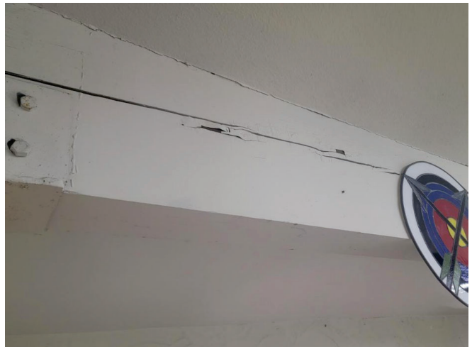
Damaged lower support beams
