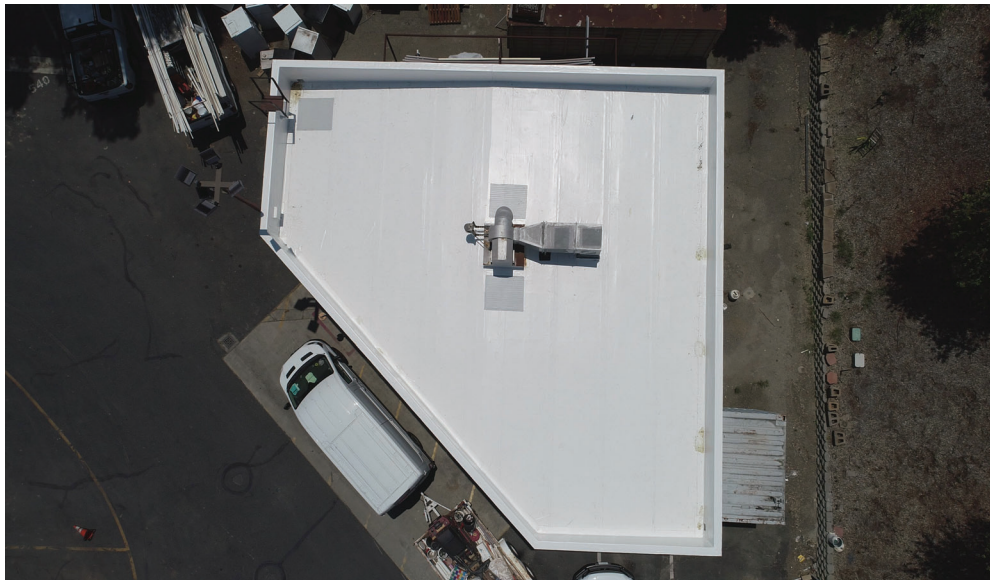
After roof replacement
