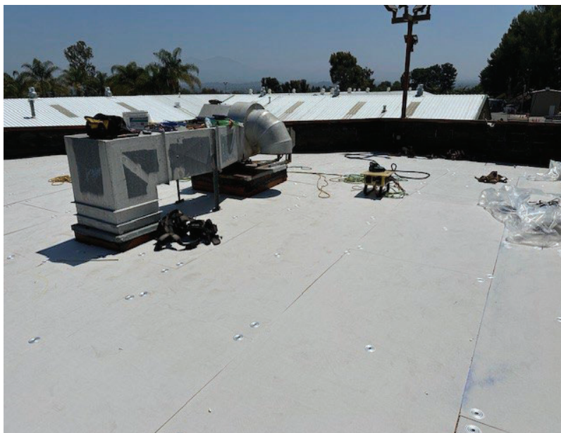
During roof replacement work
