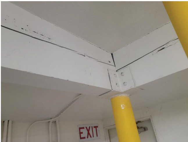
Damaged lower support beams
