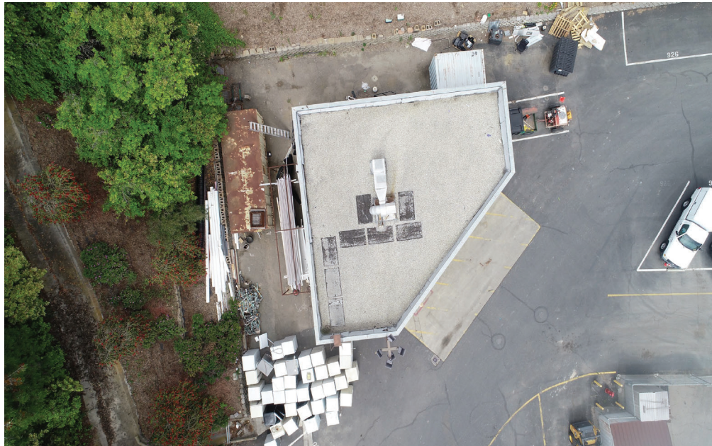
Before roof replacement
