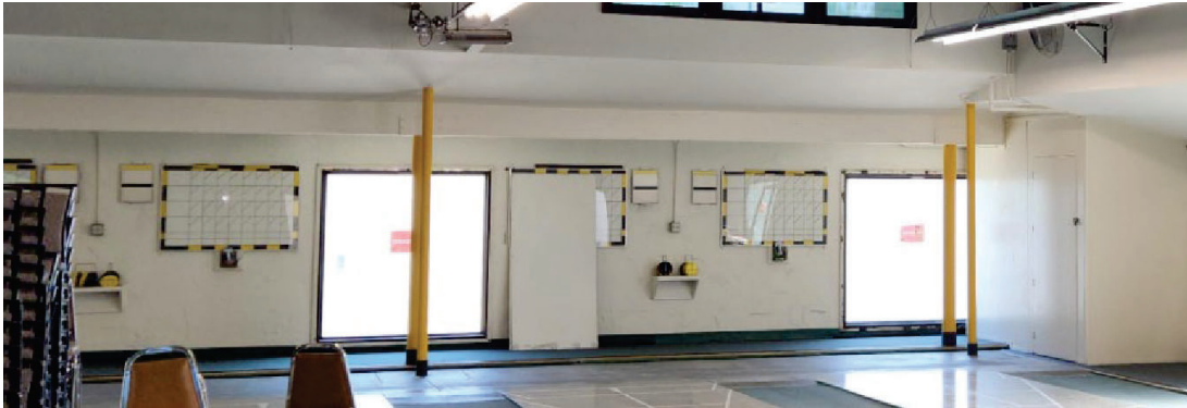
New Engineered Beams (Parallam)
